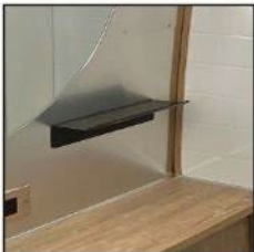
Formed Ledge-Bath Wall: 455834 MNF: Shaffer Metal Where: Aluminum wall off-set towards rear under 20" medicine cabinet mirror
