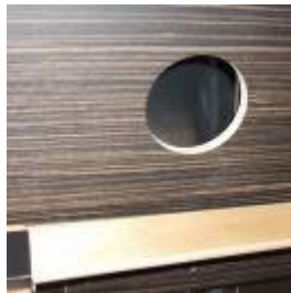
Bleeder access hole
